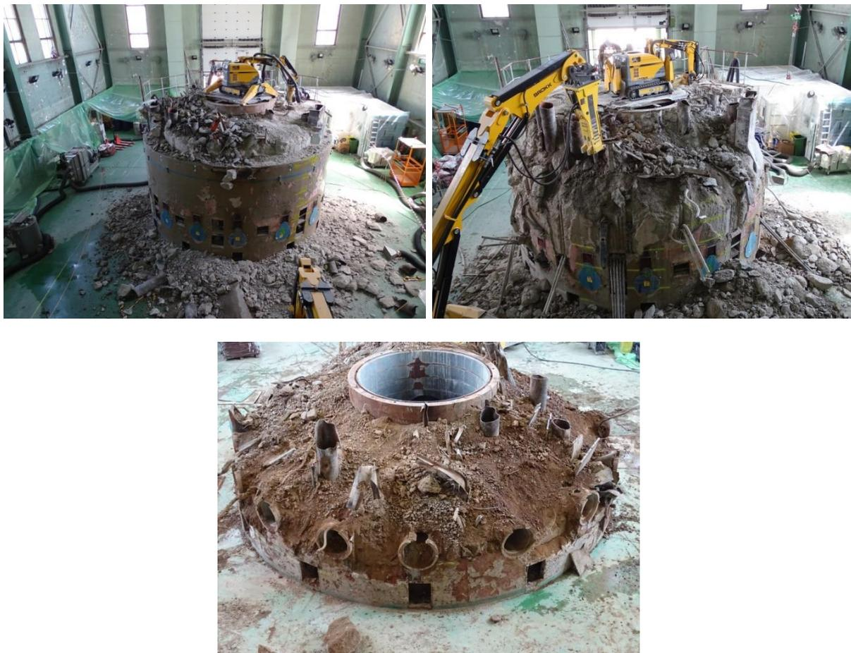
Fig.7. Stages of reactor block demolishing
