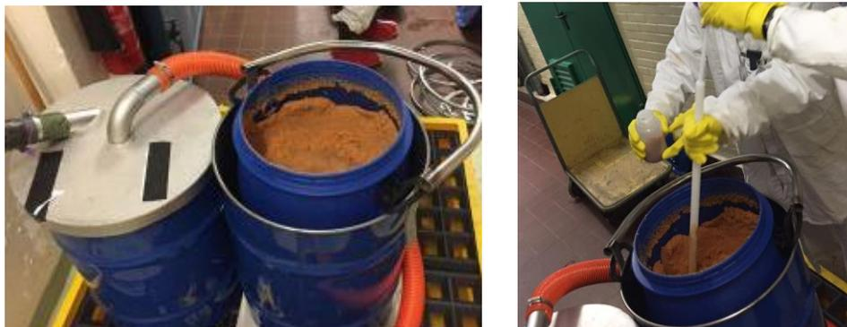
Figure 2: Replacement of the IER (filling of the containers; left) and sampling of a IER filled container (right)
