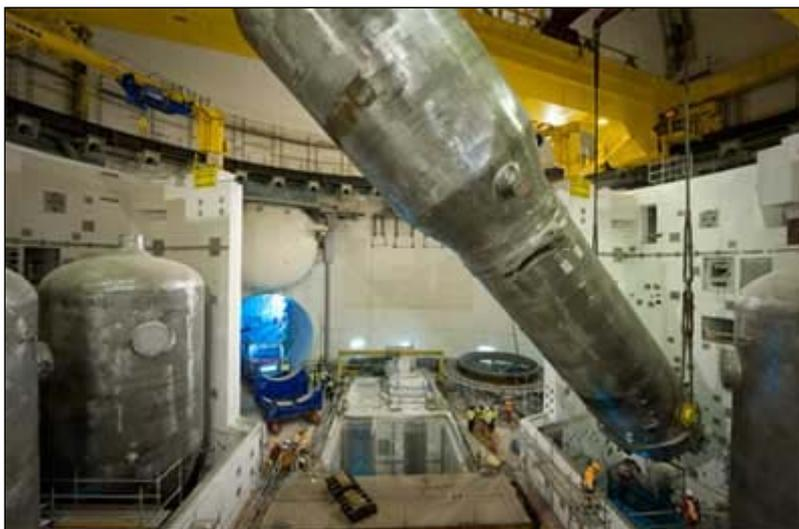
Lifting of the fourth steam generator at Olkiluoto 3 nuclear power plant (Source: TVO)
